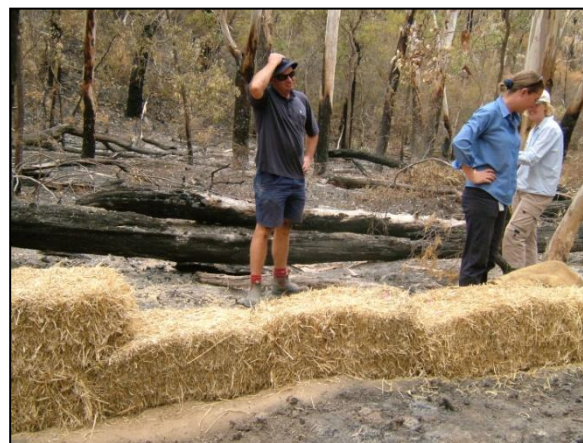
Figure 3: Installing sediment barrier traps
